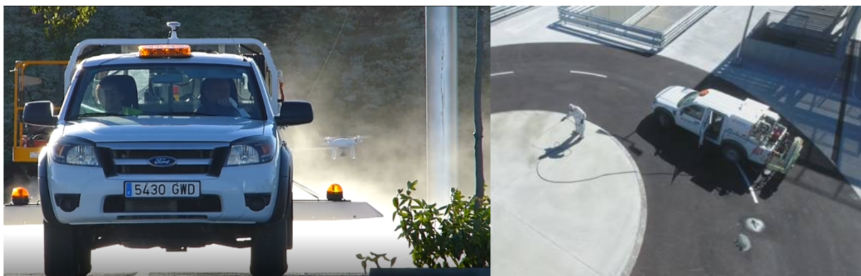
Figure 8: The automated process of utilizing PURETi coatings in main roads and surrounding areas.
